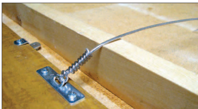
A screw eye was replaced with a steel plate and heavy wire for more reliability.
